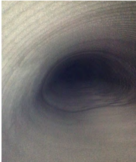
Completed arched pipelining
