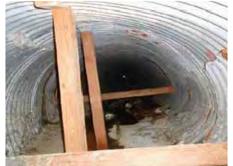
Asset owners had used timber as a temporary structural support
