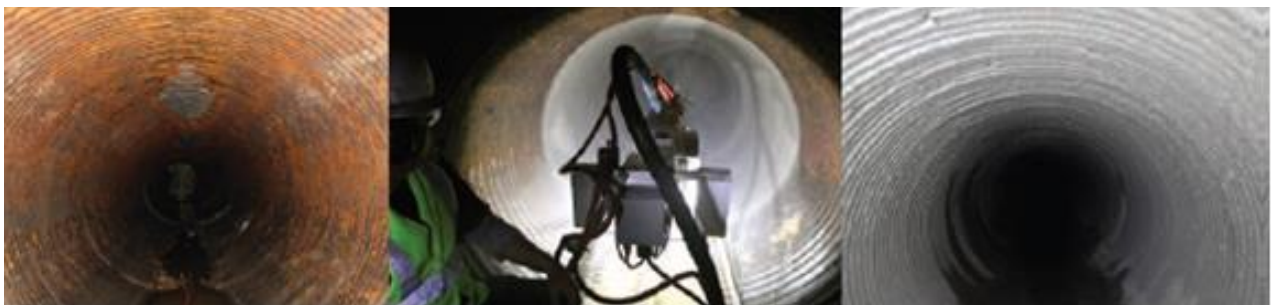
Figure 2: From left to right (a) Leaking storm water culvert (b) Centrifugal application of GeoSpray™ (c) Completed Repair 11
